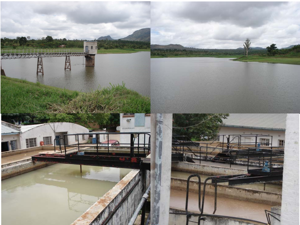
Fig. 3: Blantyre Water Board Facilities in town.
