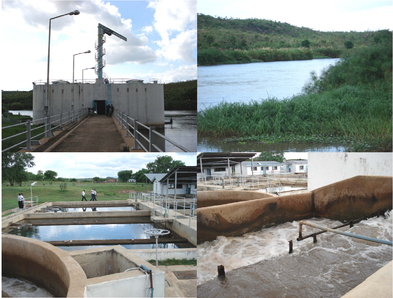
Fig. 4: Blantyre Water Board Facilities by Shire River in Chikwawa.
